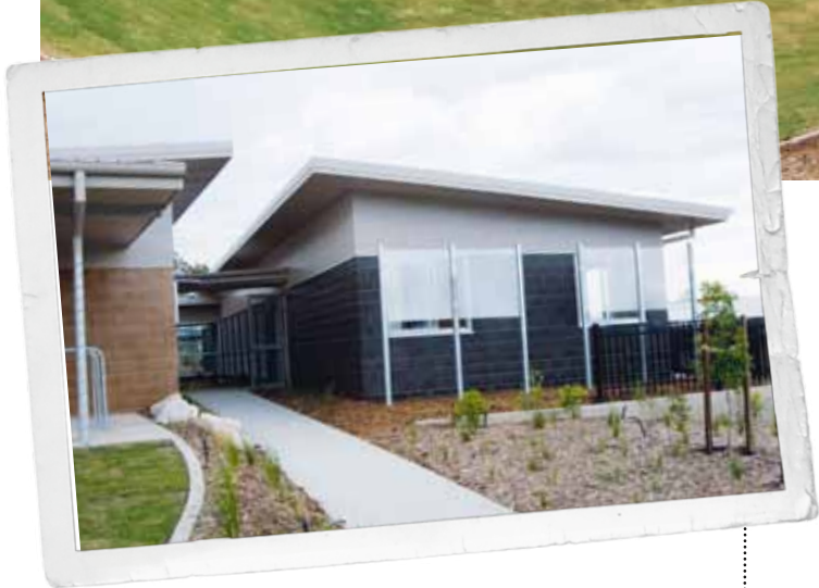
Top & inset: Passive design, natural lighting and recycling of rainwater are just three of the features of Peregian Springs State School that afford it a four Green Star rating.
